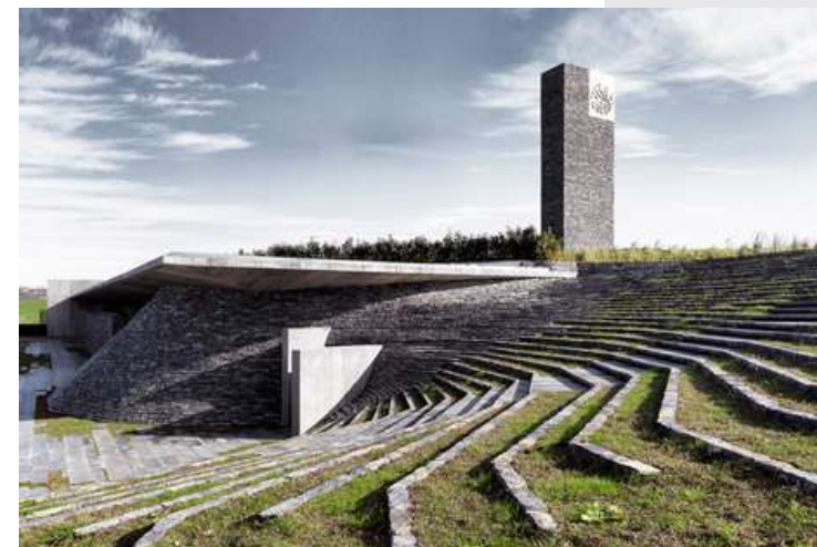
SANCAKLAR MOSQUE BY EMRE AROLAT ARCHITECTURE
