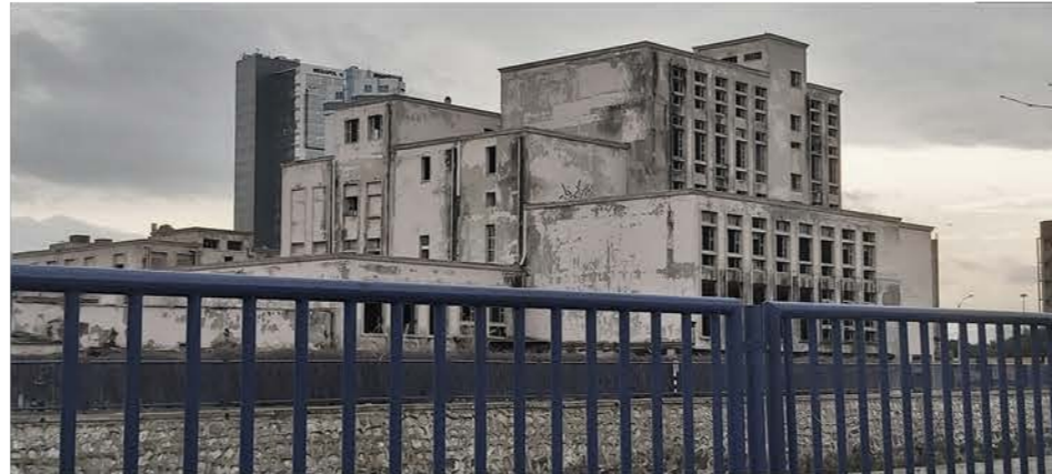
2 old factory building
