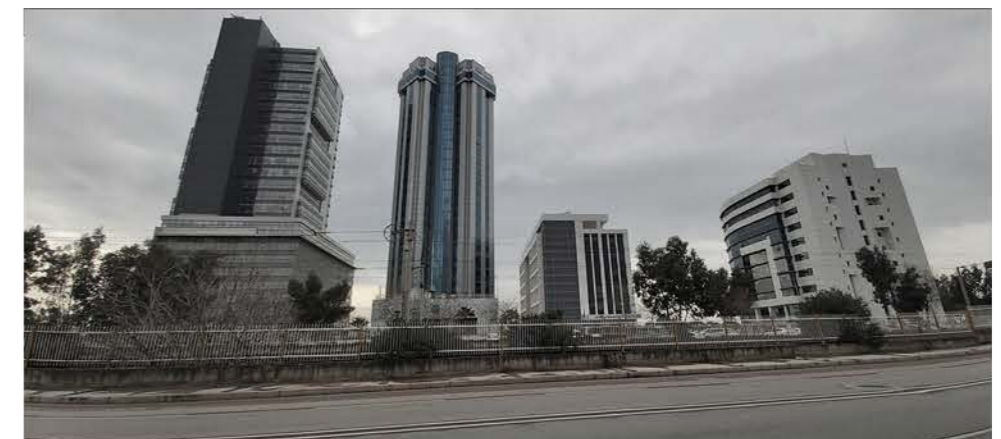
newer buildings in good condition
