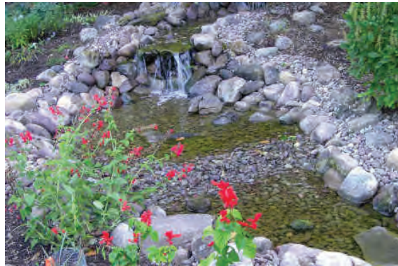
LEFT: Swale with check dams to slow the water. This creates a pleasant and aesthetically appealing ecologically sound space.
