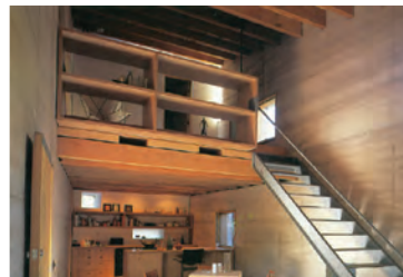
Convent Avenue Studios, Rick Joy Architects. Roof structure detail; wood beams delicately rest within rammed earth wall.
