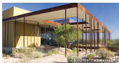
TOP: Casa Jax, Rick Joy Architects. Dwellings clad in plate steel with a ventilated air space, allowing heat to be exhausted via natural convection currents.
